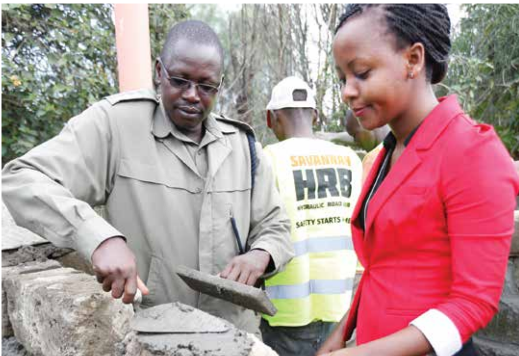
Savannah Cement project at Kitengela Police Station.
