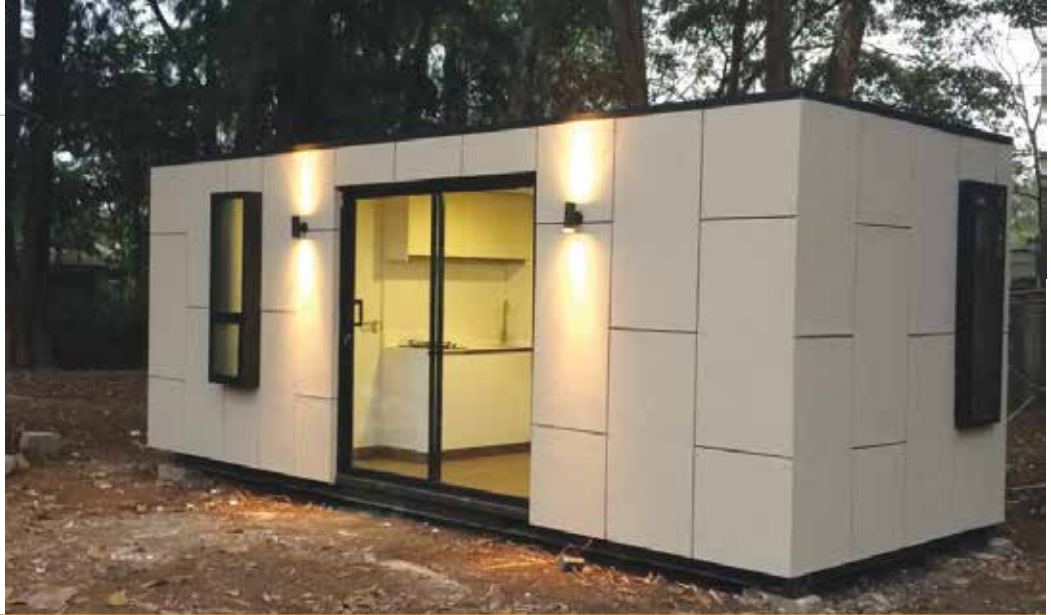
Right and below: Exterior and interior views of the Mojapod, a normal shipping container customised either into offices or homes fitted with a kitchen, bathroom and living room.
