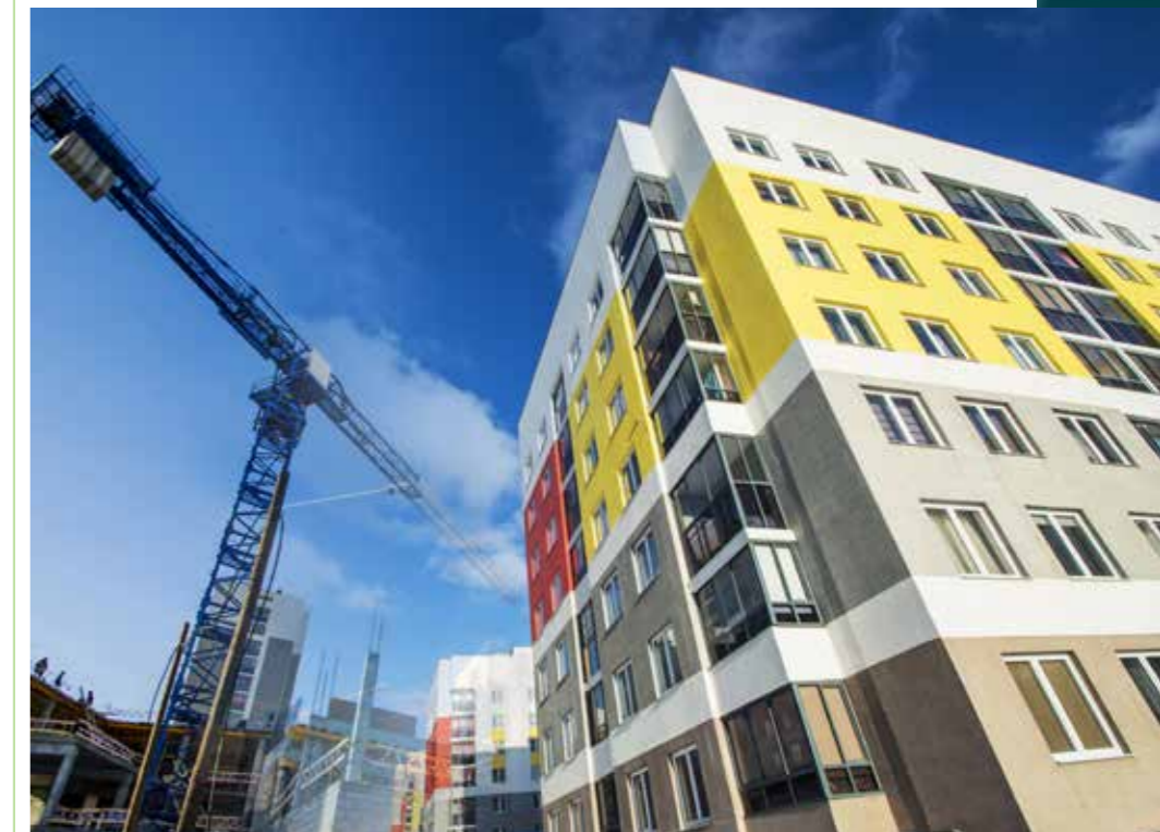
A building under construction.
